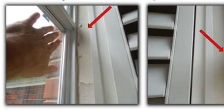
• The security sensor tabs located at the bottom portion of window frames should be sealed to help prevent moisture intrusion into the wall cavity at one or more location. It should also be noted that holes drilled in window frames for security system sensors typically voids window warranty.
