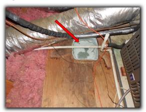
• The insulation in the overflow drain pan located under the coil housing should be removed. The insulation could clog the pan drain line and cause water to leak to the interior of the house.
