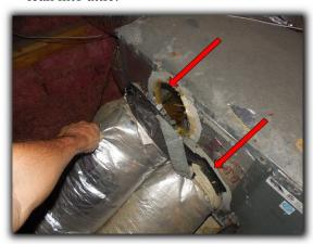
• Portion of flex duct located in attic has damaged and/or deteriorated lining. The lining keeps the insulation in place and is also used as a vapor barrier to help prevent condensation issues. Duct replacement recommended.
