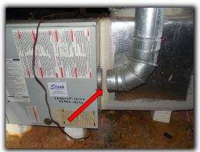
• The heater gas supply line is not equipped with a sediment trap just before the gas appliance connector. This condition does not meet current installation requirements. See correct installation at example picture below.
