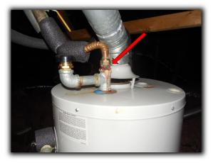
• The vent pipe is not properly mounted at the top of the water heater. This configuration will emit Carbon Monoxide into the heater compartment, which is a known <u>safety</u> hazard.
