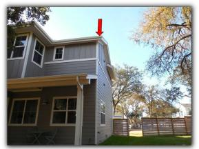
• The gutter down-spout located near front right corner house should be extended to divert runoff away from the plumbing system grinding pump control valve box.
