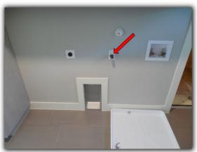
• One or more outlet was observed to have the hot and neutral conductors reversed. Find example at upstairs bedroom #3.
