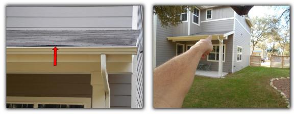
• Due to improper placement, more than one exposed shingle fastener head was observed. Find some examples at the back elevation 1st story roof starter-course.
