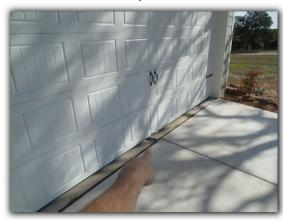
For <u>safety</u> reasons, manual locking mechanisms should be removed or disabled on overhead garage doors that are equipped with an automatic garage door opener to prevent inadvertent actuation of the opener while lock is engaged and subsequent overhead garage door damage.
