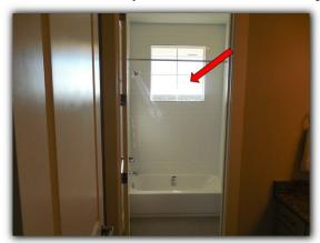
• Tempered glass (special <u>safety</u> glass) is lacking in window located at the steps landing and/or notice that the tempered glass pane has been improperly installed at wrong location or window above.
