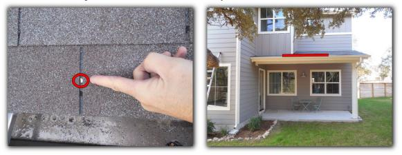
• The storm collar is not properly positioned over the roof jack at the roof level furnace flue pipe. The storm collar needs to be properly positioned and sealed to help prevent water intrusion within the roof structure.
