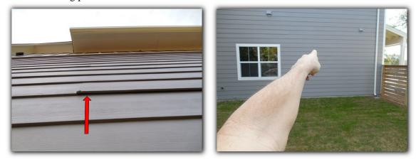
• I did not observe the installation of "Z" flashing above (2 of 3) of the back downstairs living room windows, which helps to prevent potential moisture intrusion..
