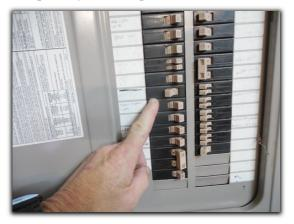
I was unable to locate a ground fault circuit interrupter (GFCI) device for the jetted tub in • master bathroom. For life/safety reasons, I advise further investigation by service specialist.
