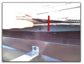
• Missing ridge shingle was observed near the back left corner house roof, which is conducive to water intrusion. A roofing contractor should be retained for remedial action.
