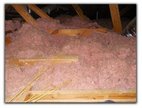
• Draft-stop and/or insulation has not been provided between the 2<sup>nd</sup> story attic flooring and the HVAC equipment platform. This condition creates un-insulated space between interior conditioned spaces of home. See example.
