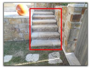
• Steps are settling and pulling away from home at one or more location. Find example at front elevation near the front left corner of house.
