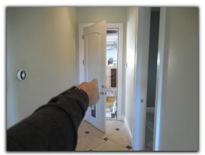
• Pet-door installation at door located between garage and home breaches door fire-separation. For life/safety reasons I advise door replacement.
