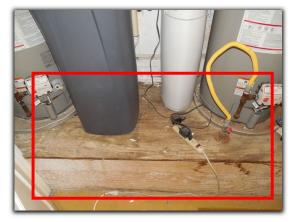
**Note:** Both water heaters are older units that may be approaching the end of its useful life. One cannot predict with certainty when replacement will become necessary. Buyer should budget for replacement. Water heaters were manufactured 2014 & 2016.
