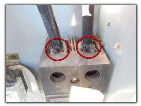
• Wire connection terminal is corroded in the main electrical panel. I advise necessary repairs by service specialist for safety reasons.
