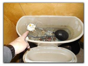
• The mount bolt gaskets are worn inside master bathroom toilet tank, which is conducive to leaks. Repair as necessary.
