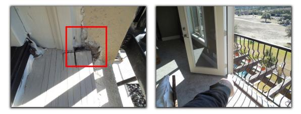
• Exterior wall claddings are not properly sealed at multiple location. These can include caulking or sealing as well as maintaining *all* joints, seams, penetrations and attachments to prevent potential water intrusion and related damage as well as proving pest and rodents a point of entry. Conditions should be self-evident to a qualified carpenter. See some examples.
