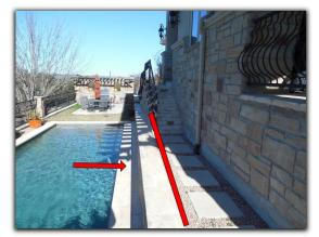
• Exterior yard steps lack handrails at more than one location, creating a potential trip hazard. Find some examples in yard near front right corner of house.
