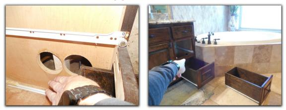
The jetted tub air switch does not properly function. It did allow me to turn equipment on, • however would not allow me to turn the equipment off after test operation. I had to shut the jetted tub system down at breaker located in garage electrical sub-panel. I advise necessary repairs by service specialist.
