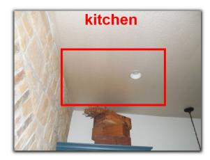
• Moisture related stains were observed on ceiling near top left corner of downstairs living room fireplace. Cause and remedy should be further investigated and corrected as necessary.
