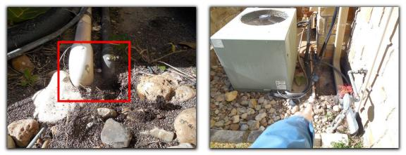
• Exposed piping at both water heaters is not protected from freeze. I advise the installation of insulation.
