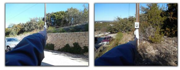
• The electrical meter and main panel are not secured to utility pole, which creates a hazardous condition. I advise necessary repairs by service specialist.
