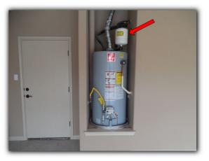
• The vent pipe is not properly positioned and mounted at the top of left side closet water heater, which will allow Carbon Monoxide into the water heater closet. For life/safety reasons. I advise necessary repairs by service specialist.
